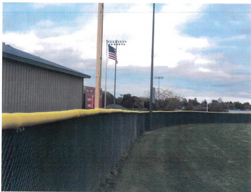
Example of outfield fence with plastic cap.
