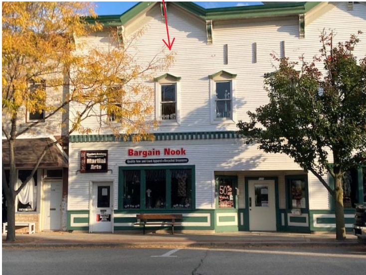
Present location - upstairs
