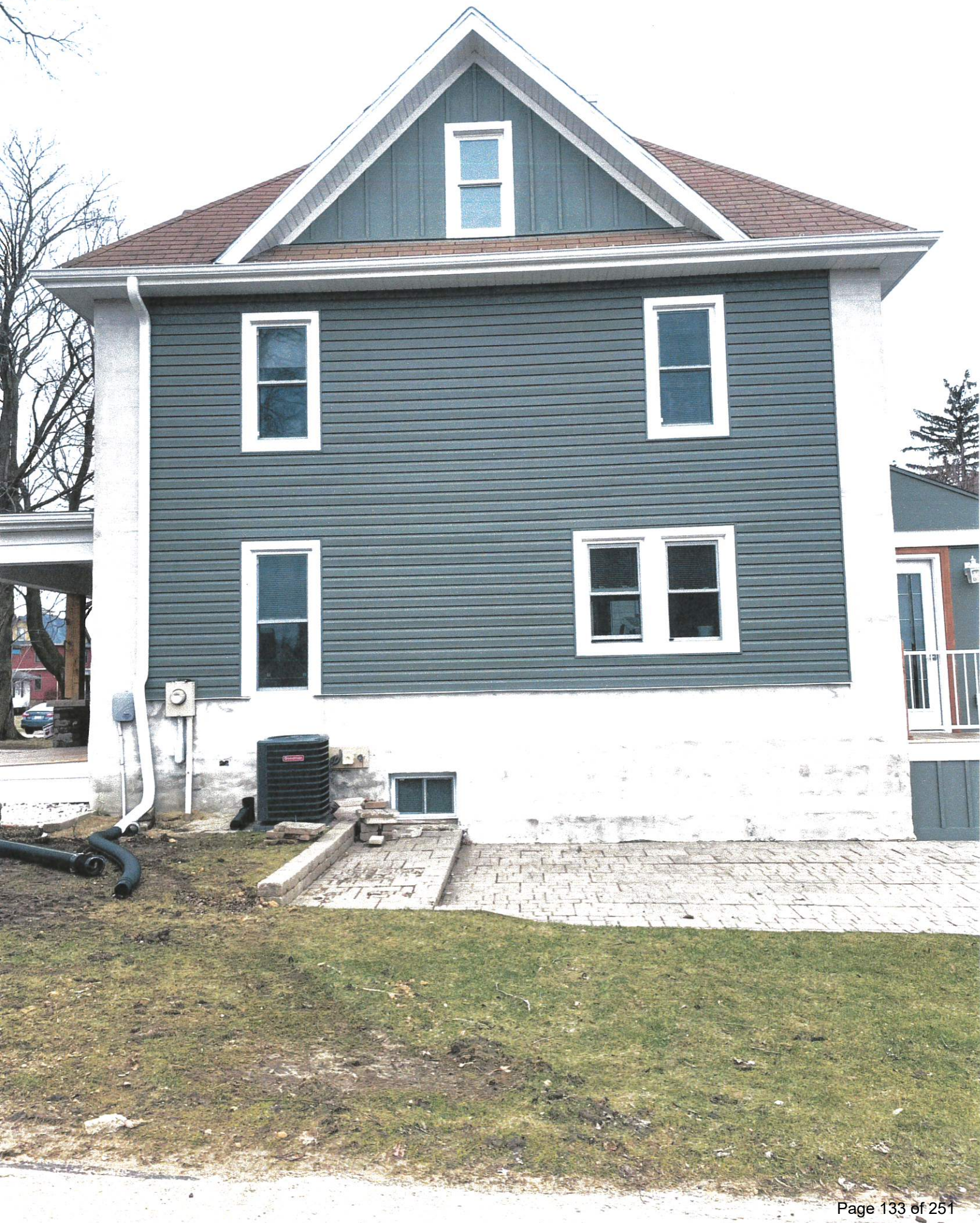
BEFORE- East Elevation
