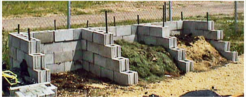
Concrete Block Three-Bay
