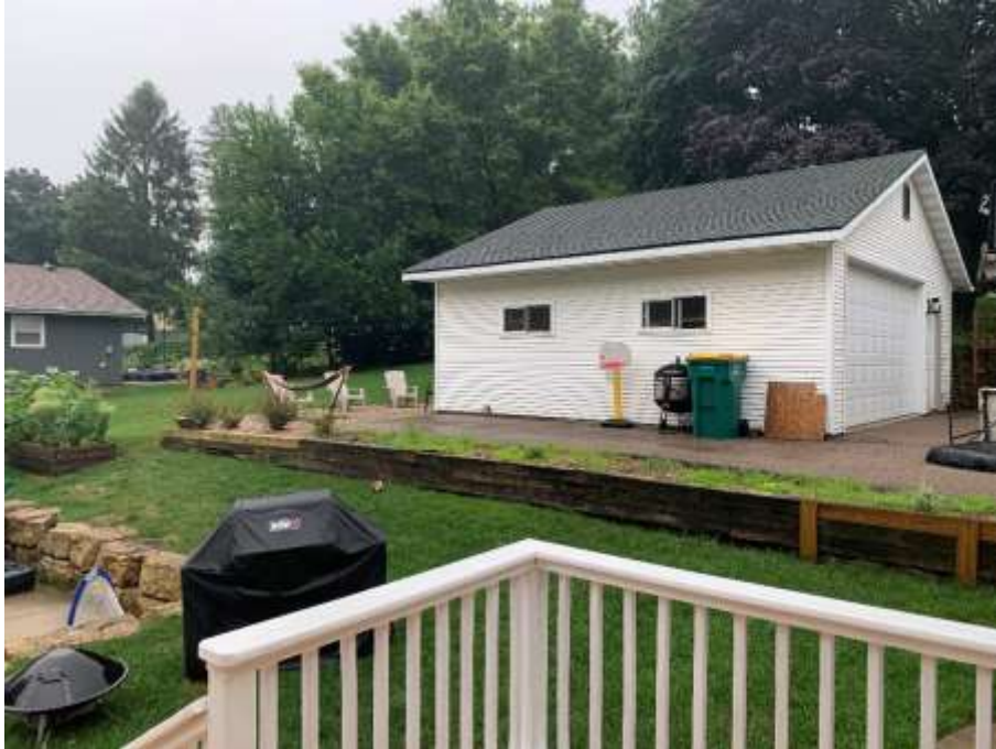
Image 1: Photo taken facing southeast at the failing retaining wall visible to all park goers. The lowest timber layer is completely rotted. The wall is tipping and does not stand vertical.
