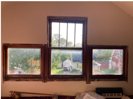
East Interior Windows -1 double hung -2 fixed frame
