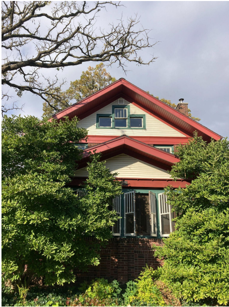
East Exterior Windows (sidewalk)
