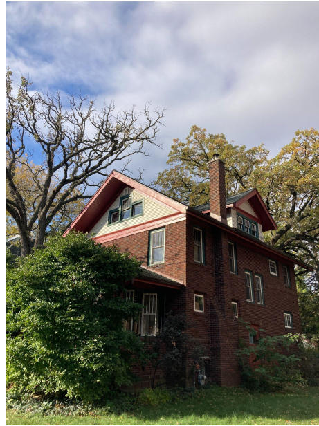
North Exterior Windows (sidewalk)
