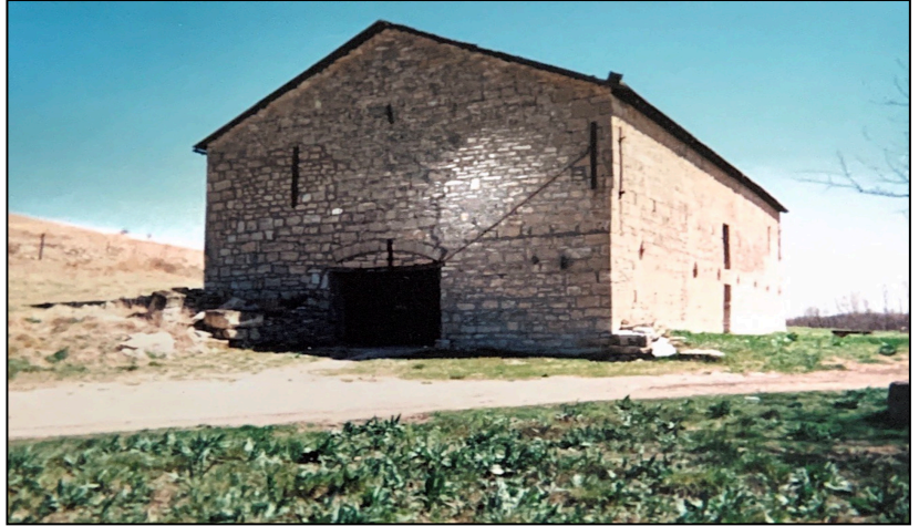
Figure 5. Post Rock Structure. Source: Kansas Historical Society
