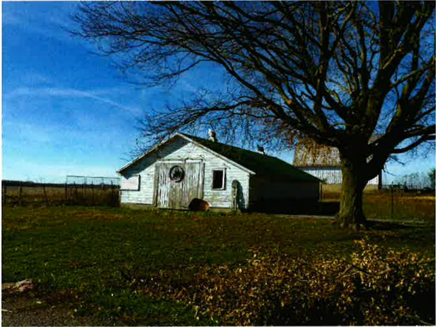
Photo 5. Livestock Shed, camera facing southwest.
