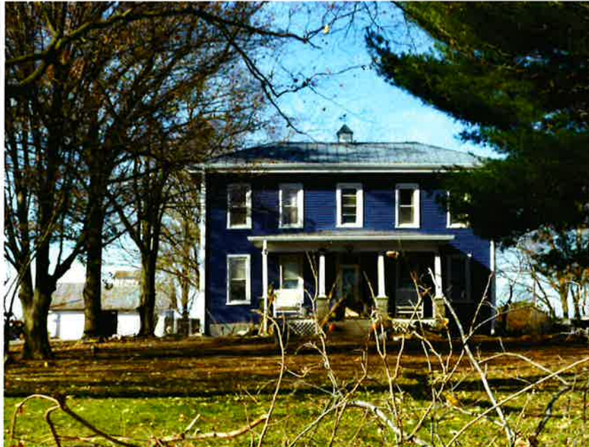
Photo 1. House, camera facing west.
