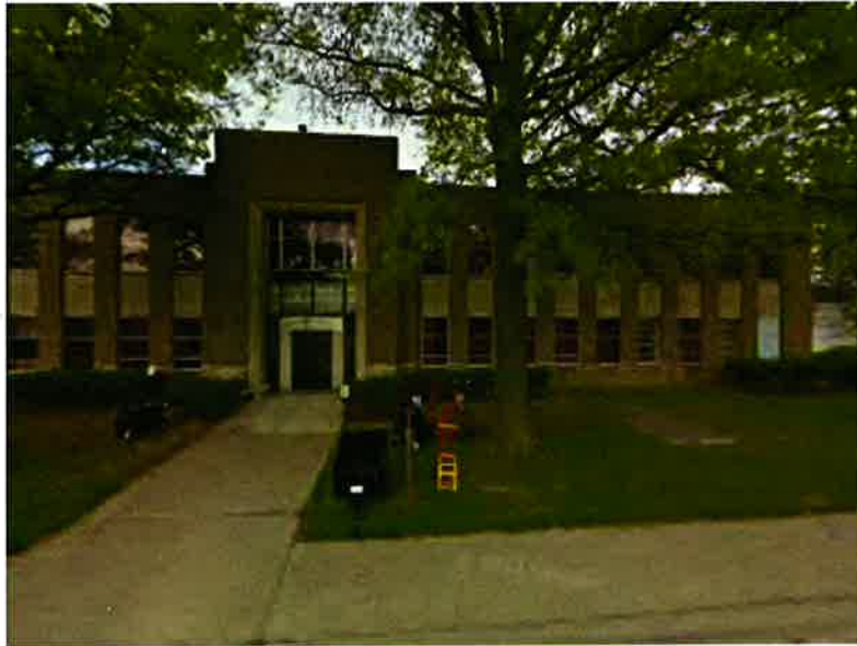
Photo 21. Lehn & Fink, camera facing east (image from Google Earth).
