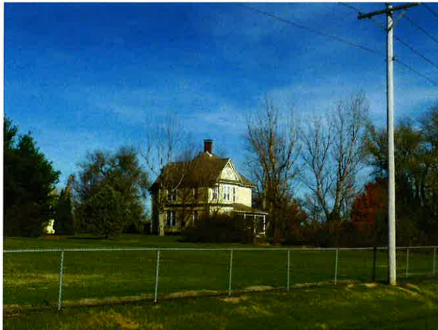
Photo 16. House, camera facing northeast.
