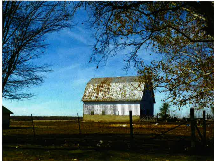
Photo 4. Barn, camera facing southwest.
